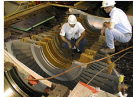
Steam Turbine Internals Alignment
