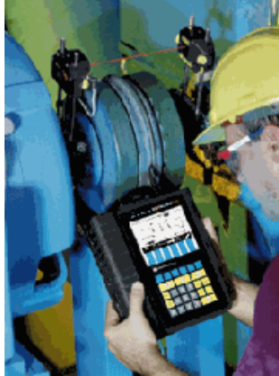
Laser shaft alignment of a feed water pump
