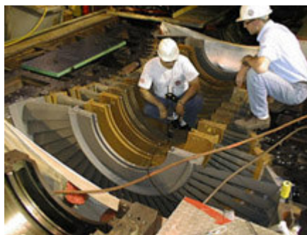
Steam Turbine Internals Alignment
