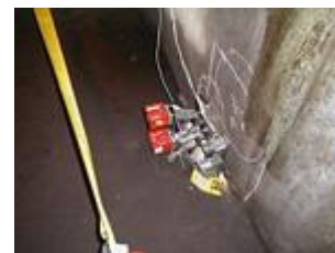
Laser and Strain gauge measurement of steam turbine foundation pedestal movement in Ohio.
